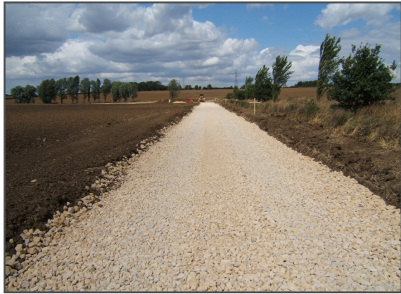
Plate 6.3 - Typical New Site Access Track
