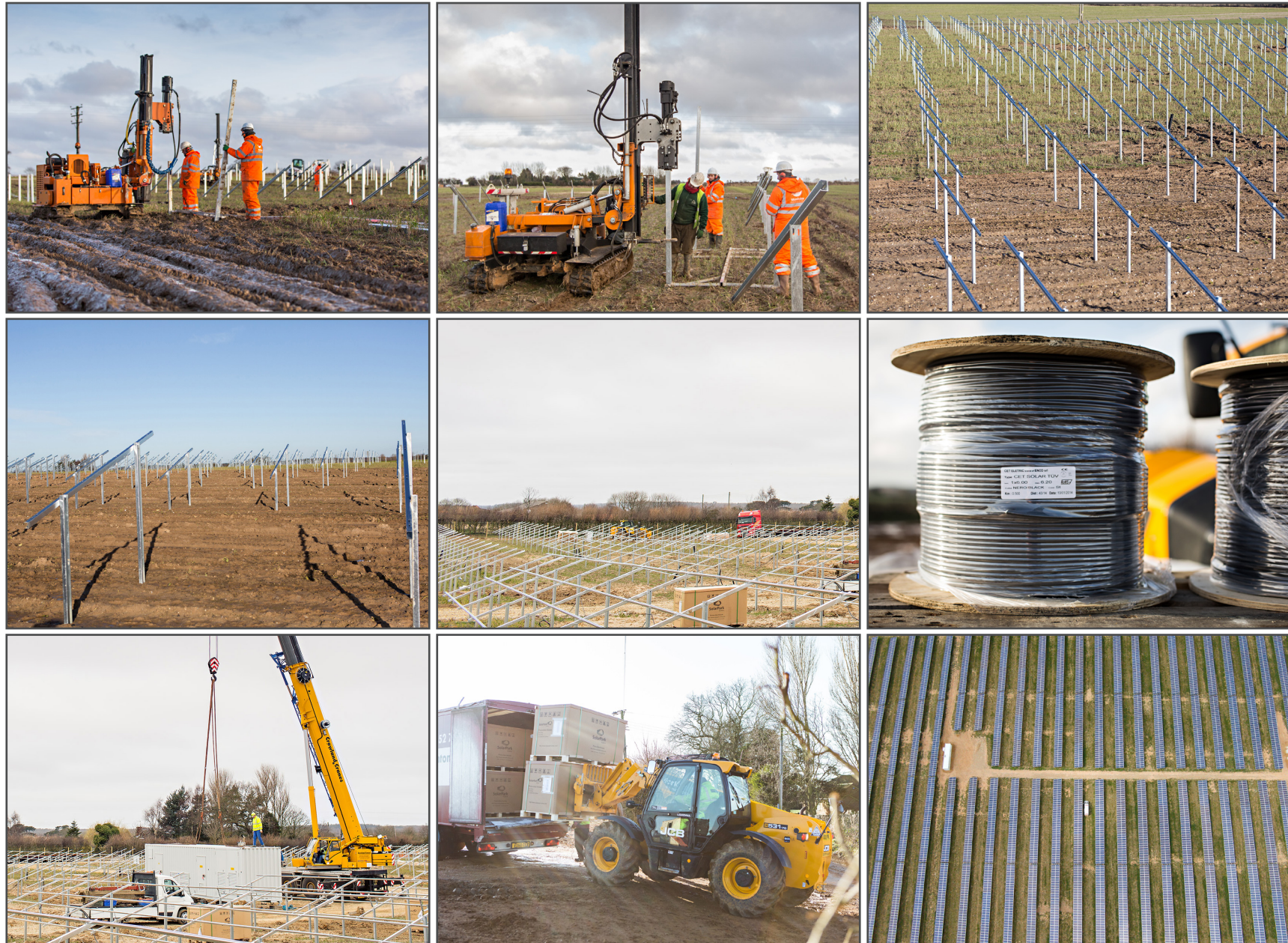
Plate 7.1 - Photographic Sequence of Construction Process
