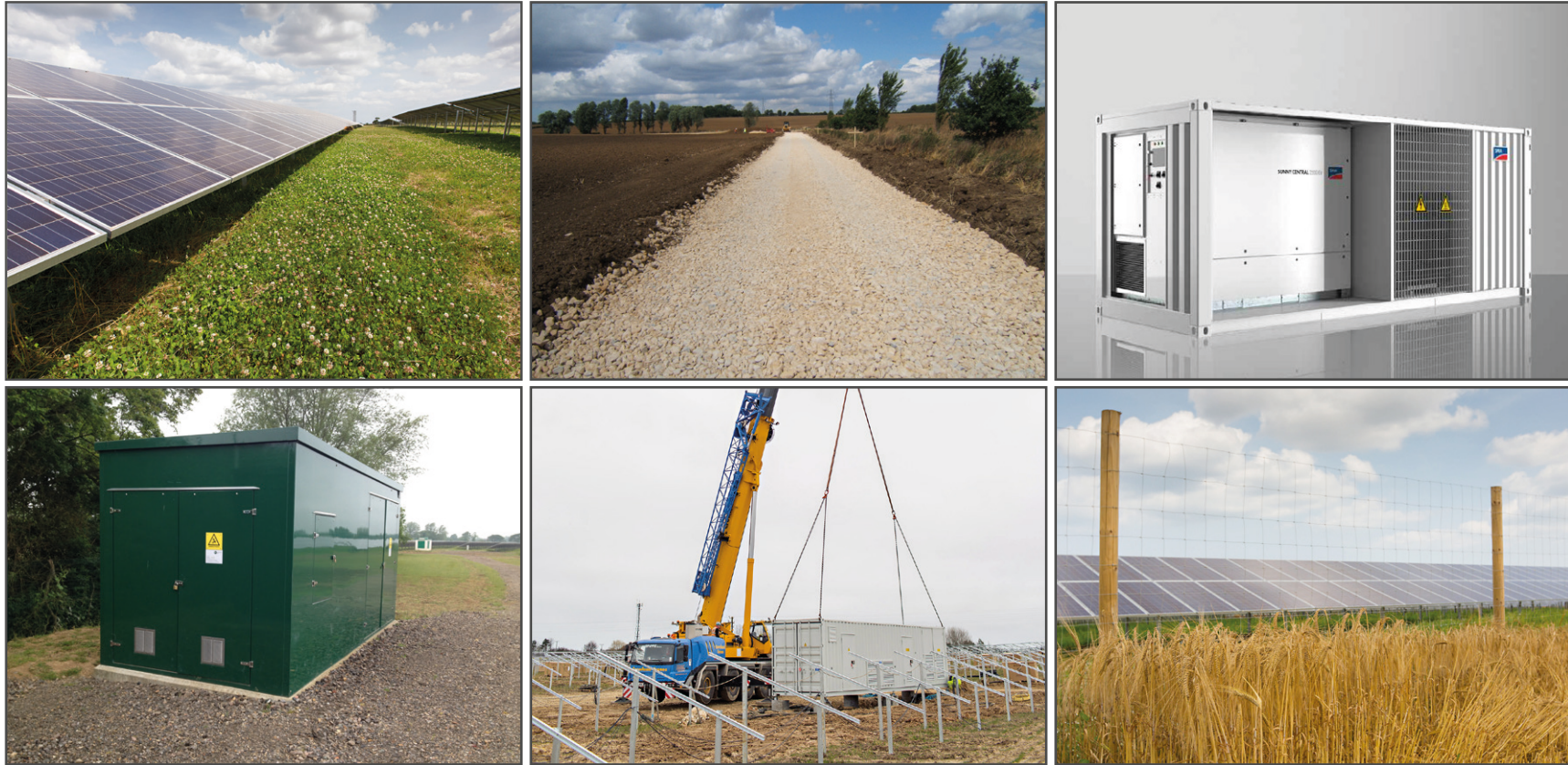
Plate DA.1 - Typical Solar Farm Infrastructure Appearance (colour finish to be agreed with Ashford Borough Council) - clockwise from top left: installed panels; typical site track; typical inverter/transformer unit; typical cabinet; construction works; typical site fencing and installed panels.
